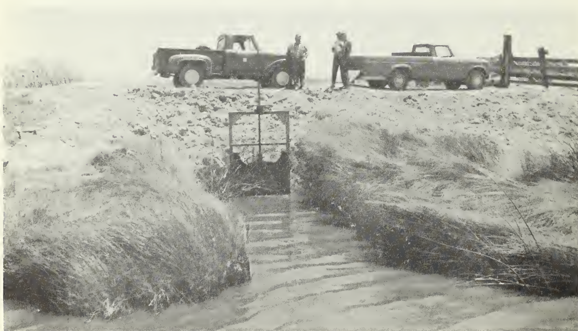
Photo 7. Above type of water control structure installed.
